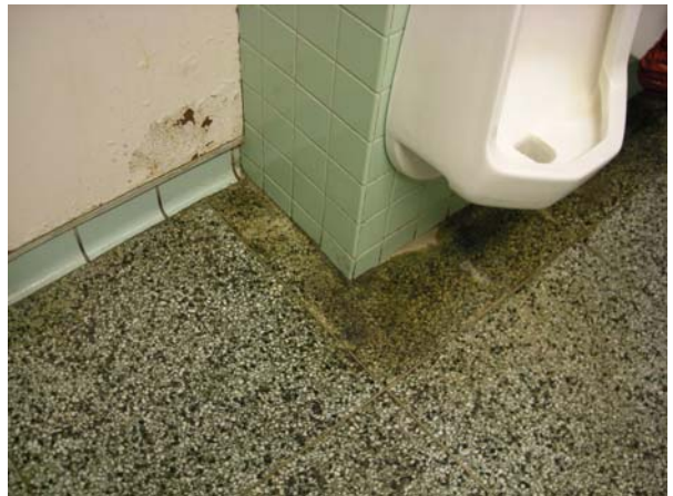
Damaged Terrazzo and Access Panel
