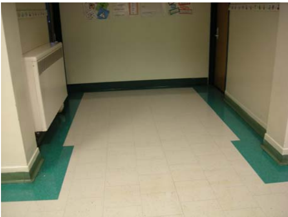
Unit Ventilator in Corridor
