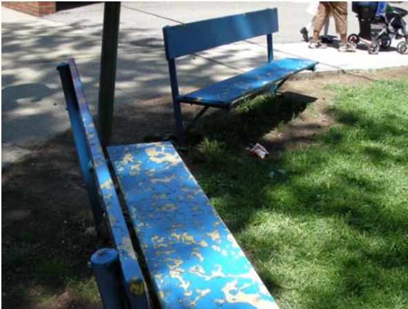
Benches Needing Replacement
