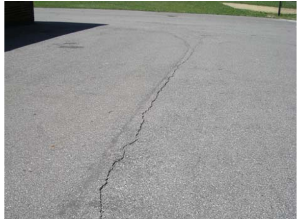
Typical Asphalt Condition
