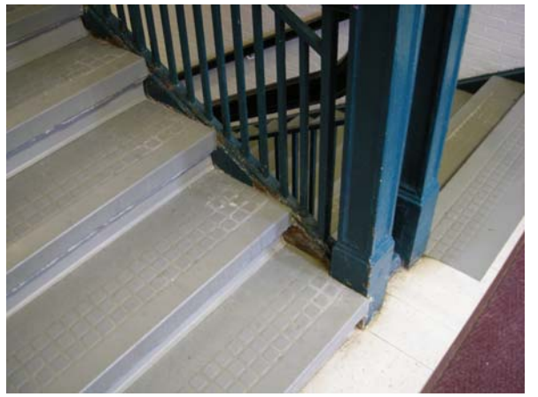
Staircase Corrosion
