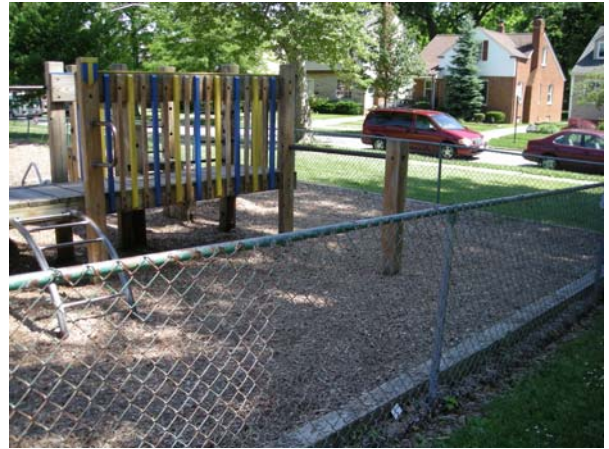
Typical Condition of Site Fence
