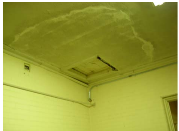
Plaster Damage in Basement
