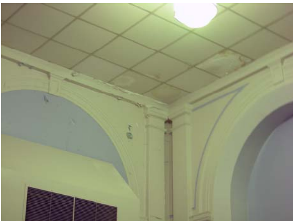
Plaster Damage in Cafeteria
