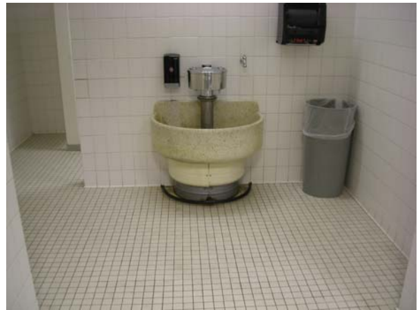
Restroom Fixtures and Accessories
