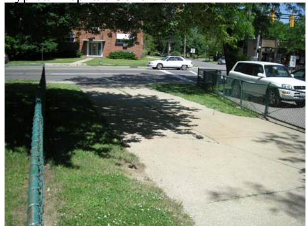
Concrete Needing Replacement
