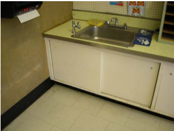
Obsolete Casework - Kindergarten
