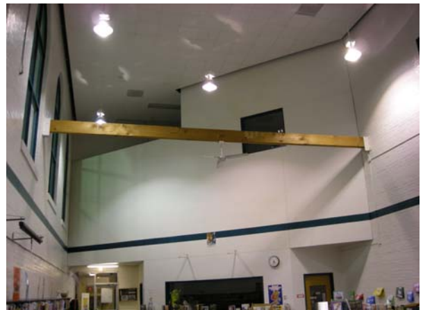
Ceiling Fans in Media Center
